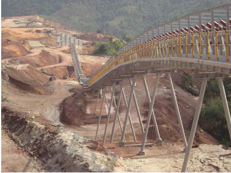
Steel work for the one-kilometre overland conveyor is complete
