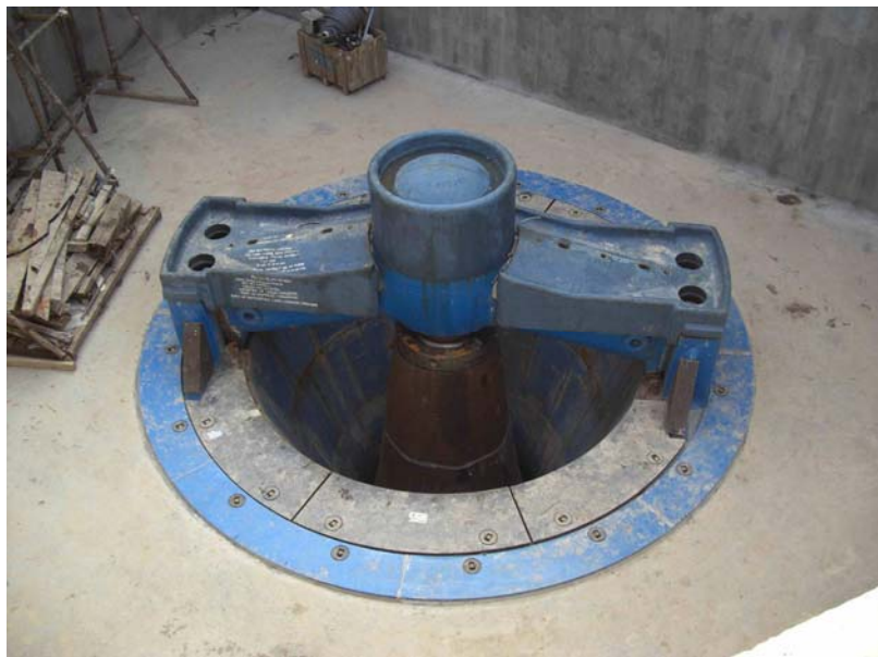
Primary crusher installed
